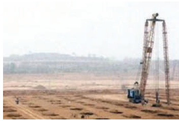
Fig. 5 (a): Construction example of dynamic compaction.
